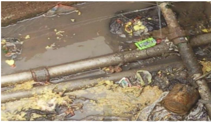
Plate 2: water pipes in sewers
